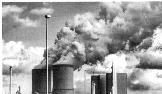
Steel Building Industry Factory Power Plant
